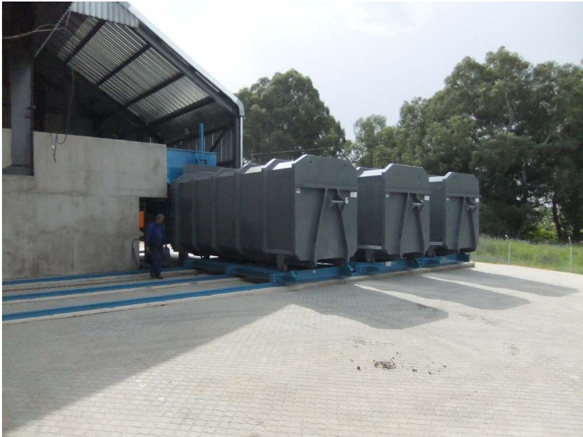
Figure 3-23: Paarl Solid Waste Transfer Station
