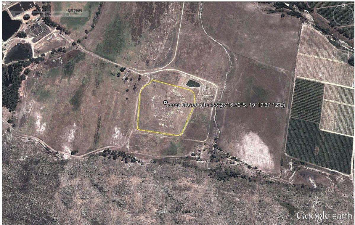
Figure 3-21: Ceres Closed Landfill
