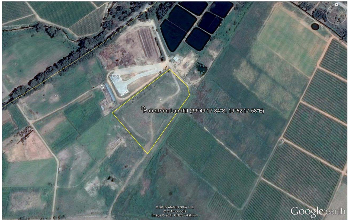
Figure 3-20: Robertson Rehabilitated Landfill
